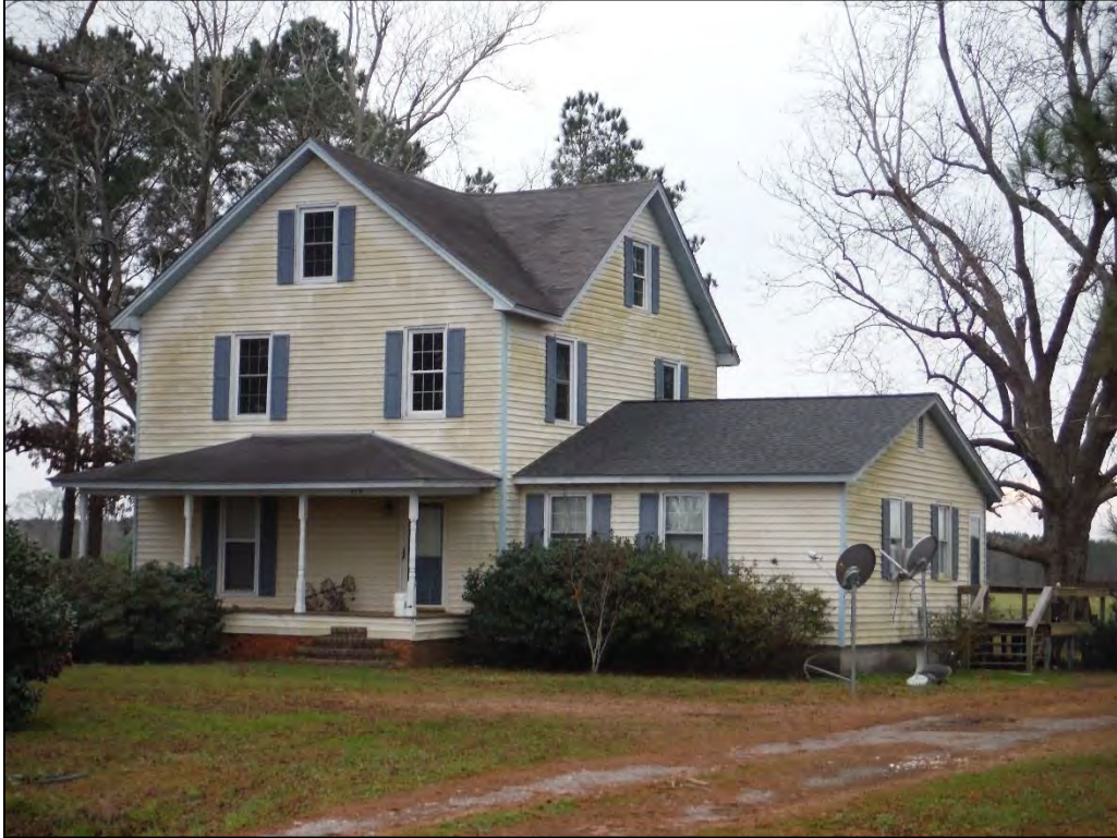
Figure 16. Ben Manning House (HY0183) at 826 Sladesville Road, facing southwest.
