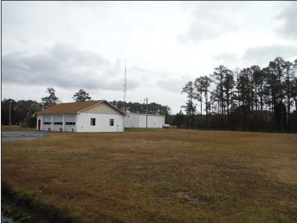
Figure 84. Sladesville School House property, facing southeast.
