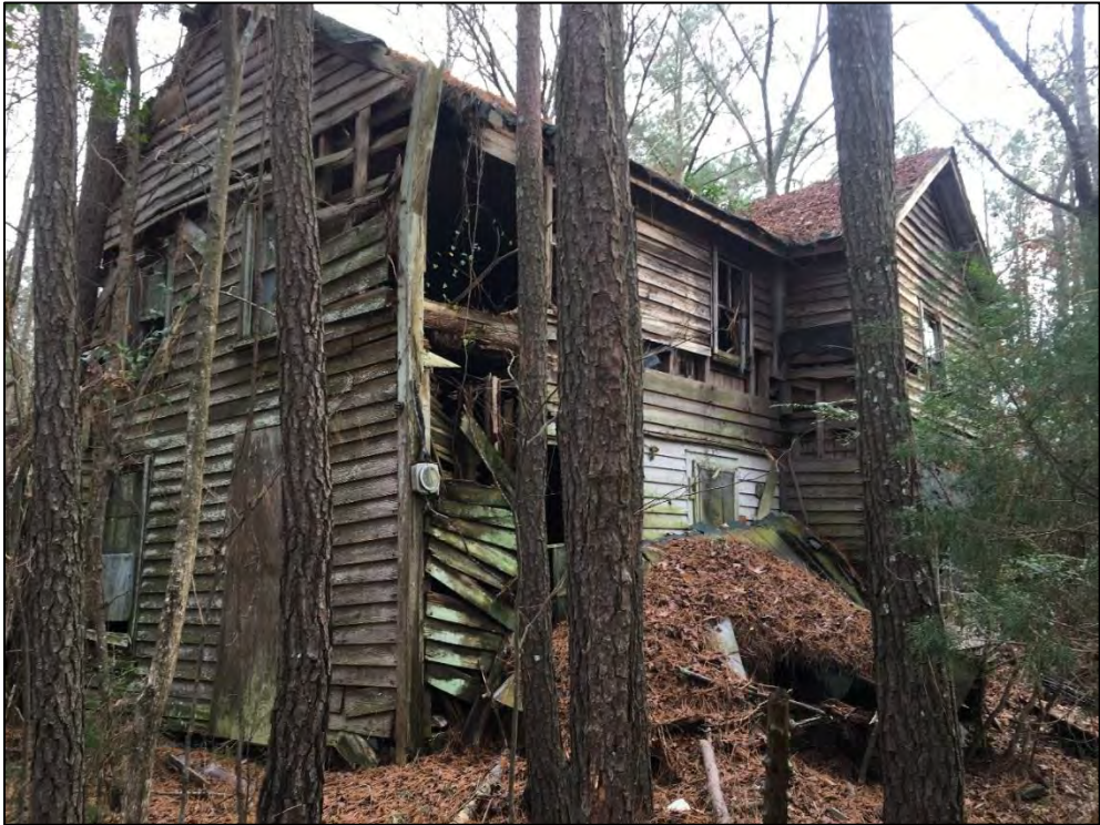
Figure 57. Jarvis-Elixson House, facing southeast.
