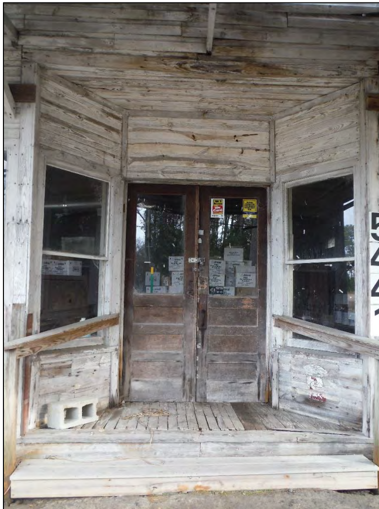
Figure 26. Detail of entryway of the Napoleon Sears Store, facing east.
