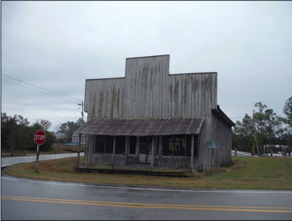
Figure 30. J. Montier Hall Store and Warehouse (NSN), 11 White Plains Road, facing east.
