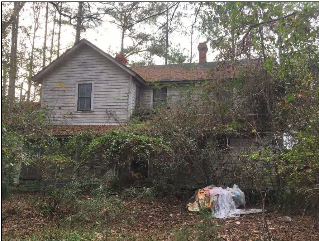
Figure 72. Jarvis-Sears House, facing west.
