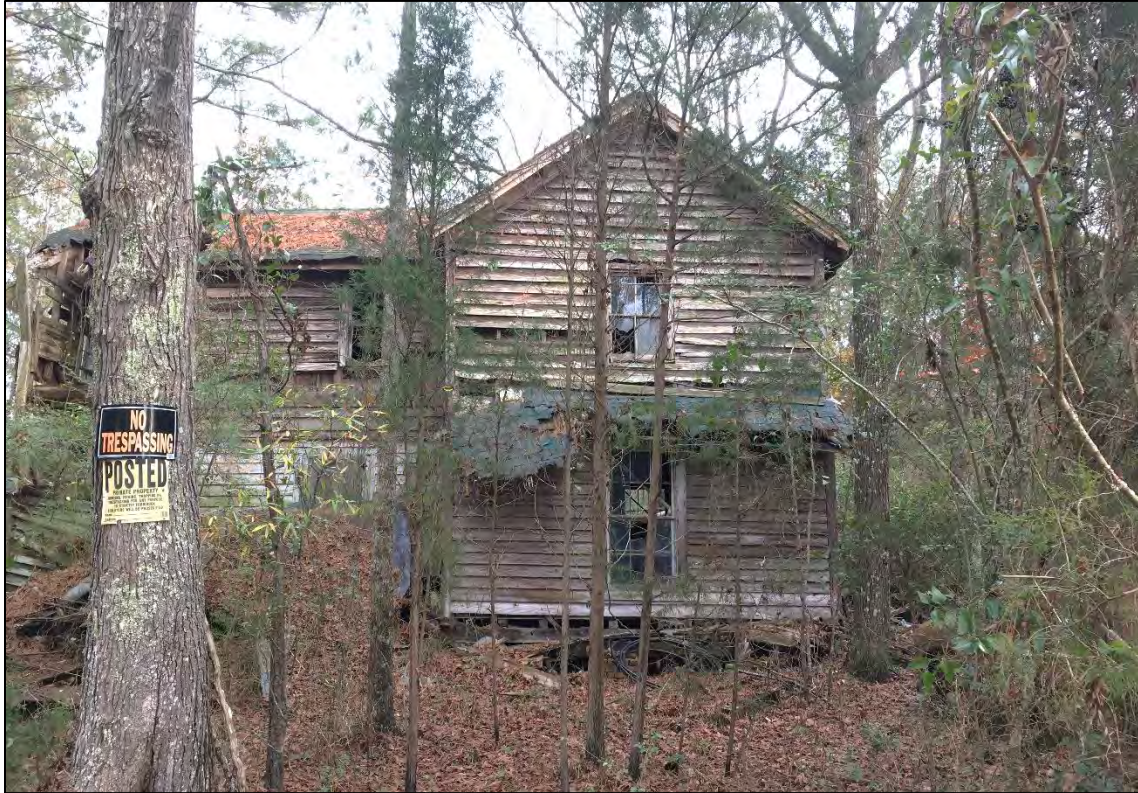
Figure 56. Jarvis-Elixson House, facing east.
