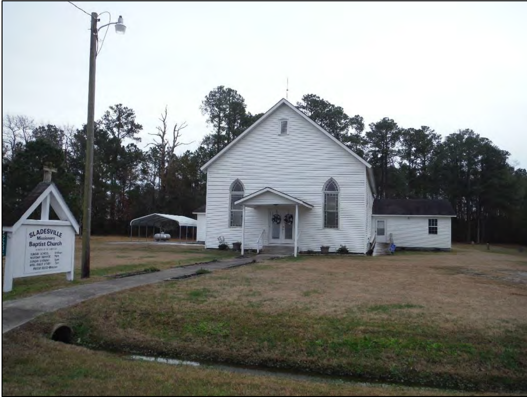
Figure 50. Sladesville Missionary Baptist Church (HY0186), facing south.
