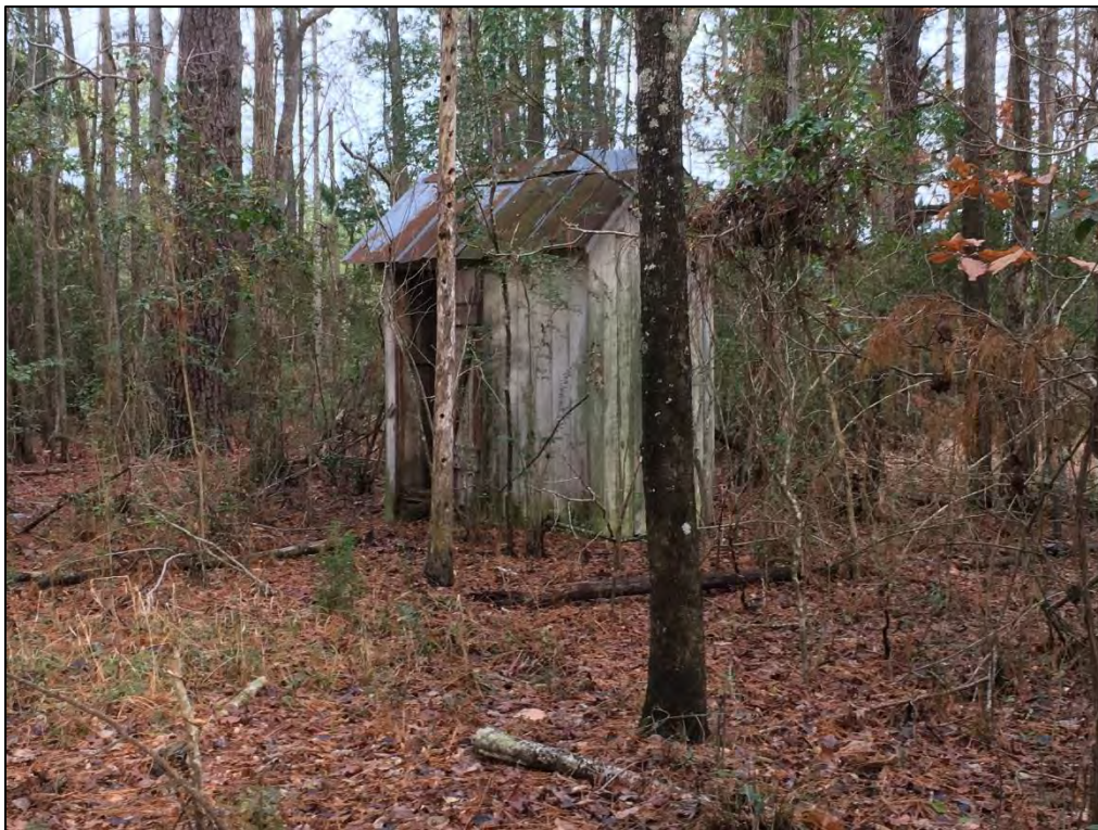
Figure 80. Storage building on the Jarvis-Sears House property, facing northwest.
