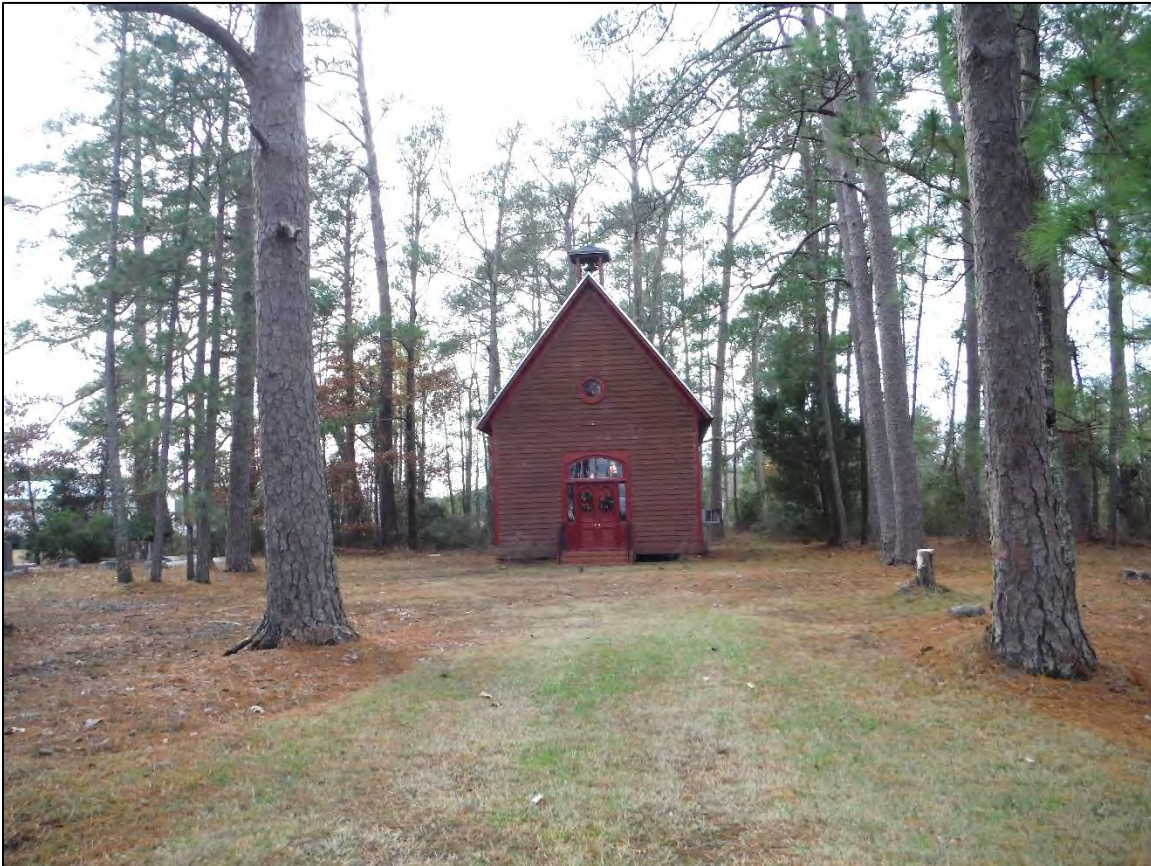
Figure 35. St. John's Episcopal Church, facing west.
