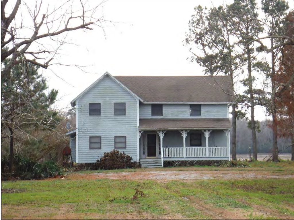
Figure 19. Benson-Howard House (HY0166), 22176 US 264, facing south.
