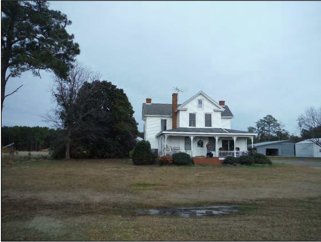
Figure 14. John Ruffin House (HY0148) at 1324 Loop Road, facing northeast.
