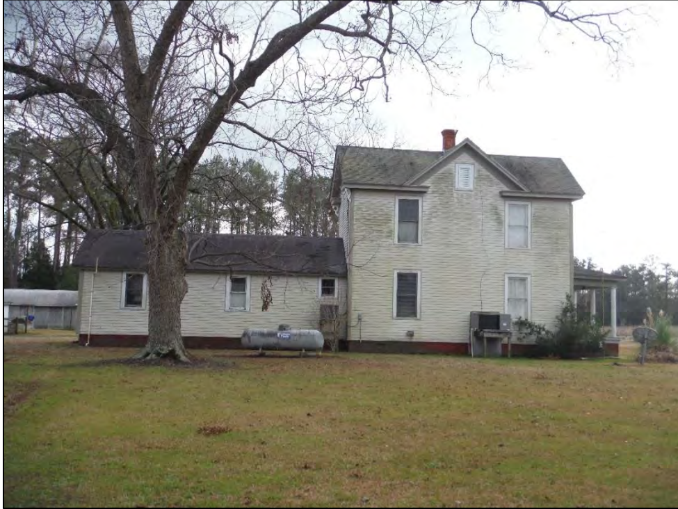
Figure 8. Gratz Credle House, facing south.
