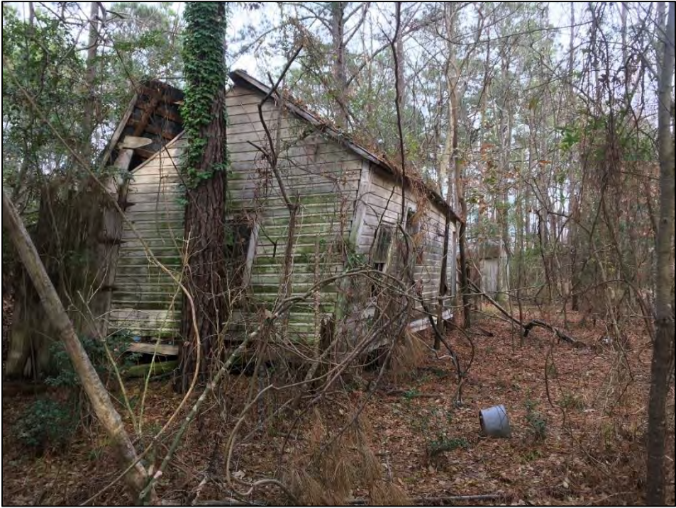
Figure 78. Storage building on the Jarvis-Sears House property, facing northeast.
