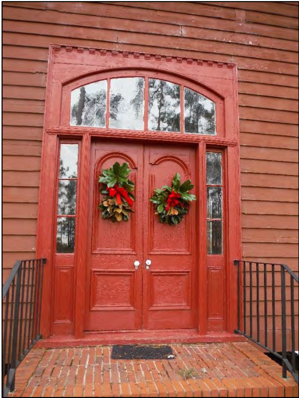
Figure 37. Detail view of front entry doors, St. John's Episcopal Church, facing west.
