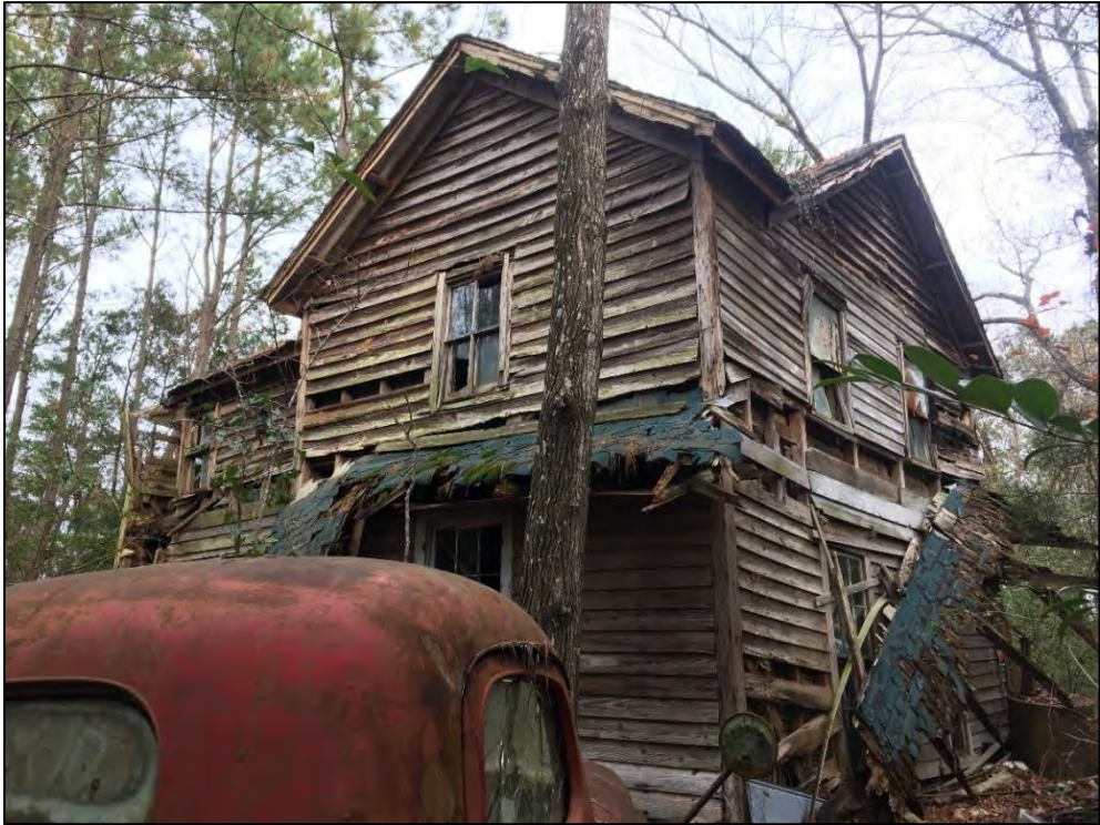
Figure 58. Jarvis-Elixson House, facing northeast.
