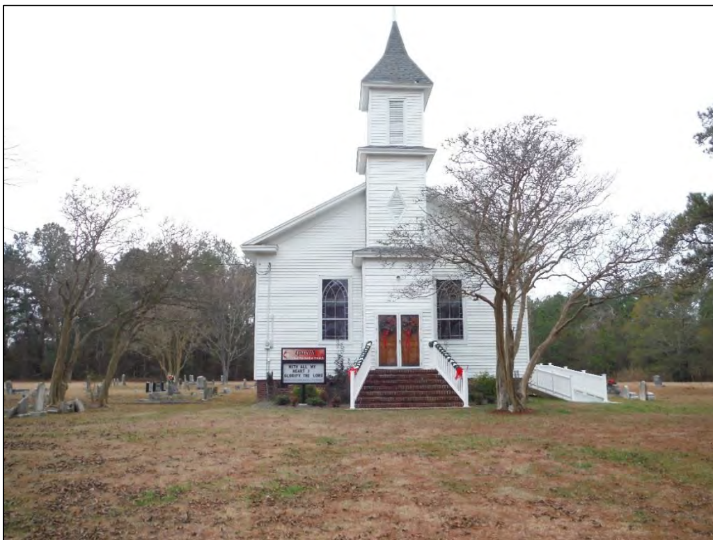
Figure 49. Epworth Methodist Church (HY0185), facing east.
