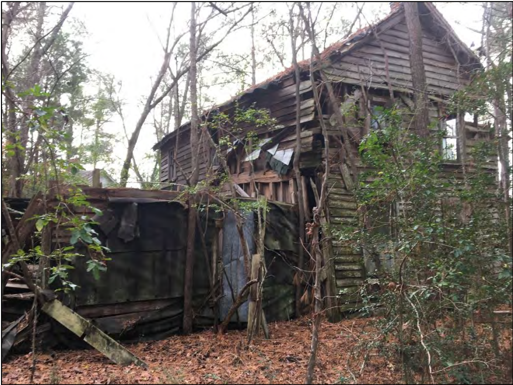
Figure 61. Jarvis-Elixson House, facing southwest.
