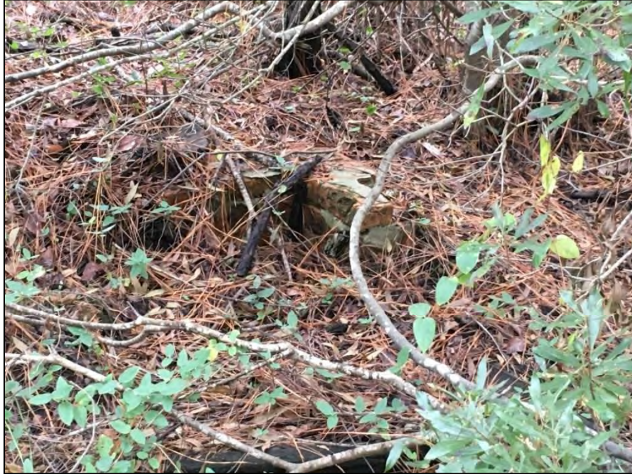
Figure 90. Brick foundation on unnamed House property, facing east.
