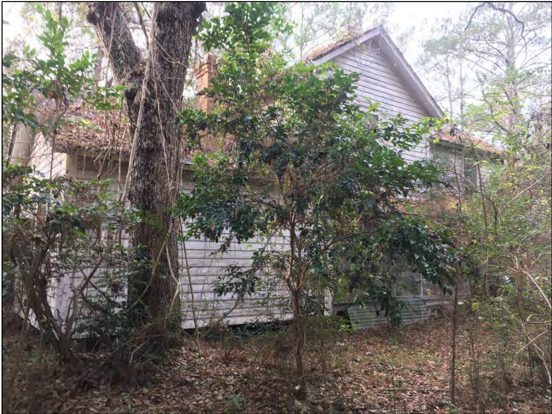
Figure 74. Jarvis-Sears House, facing northwest.
