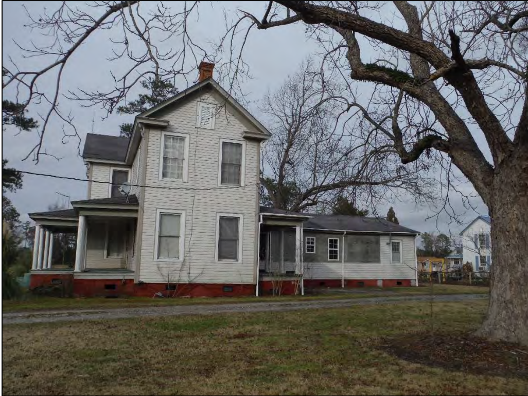
Figure 6. Gratz Credle House, facing north.
